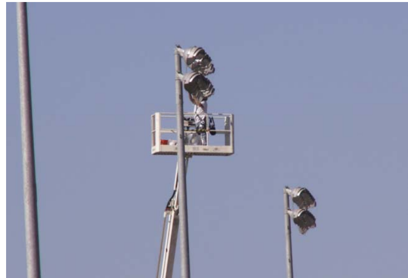
Replacing damaged reflector lens
