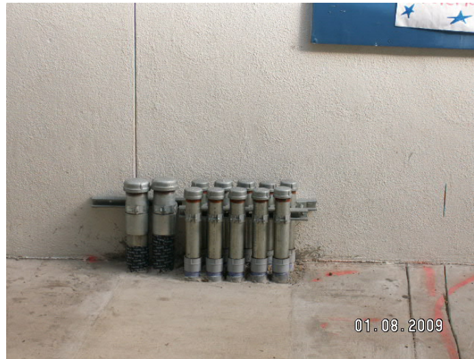
New spare future conduits for use as Signal & Data runs
