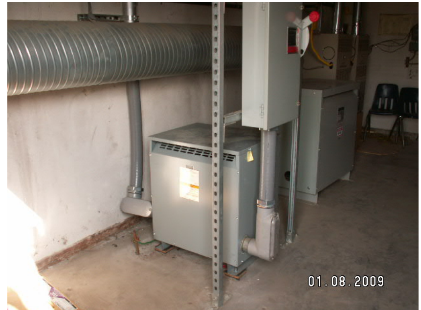
New transformer by change order in Building #25
