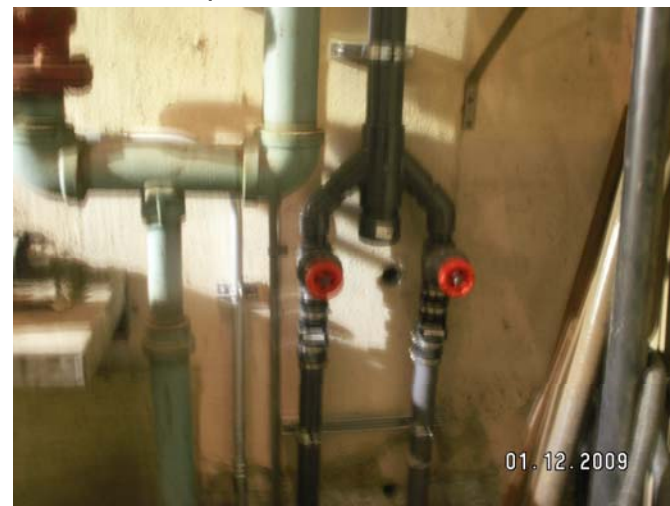
Discharge manifold for interior sump pumps
