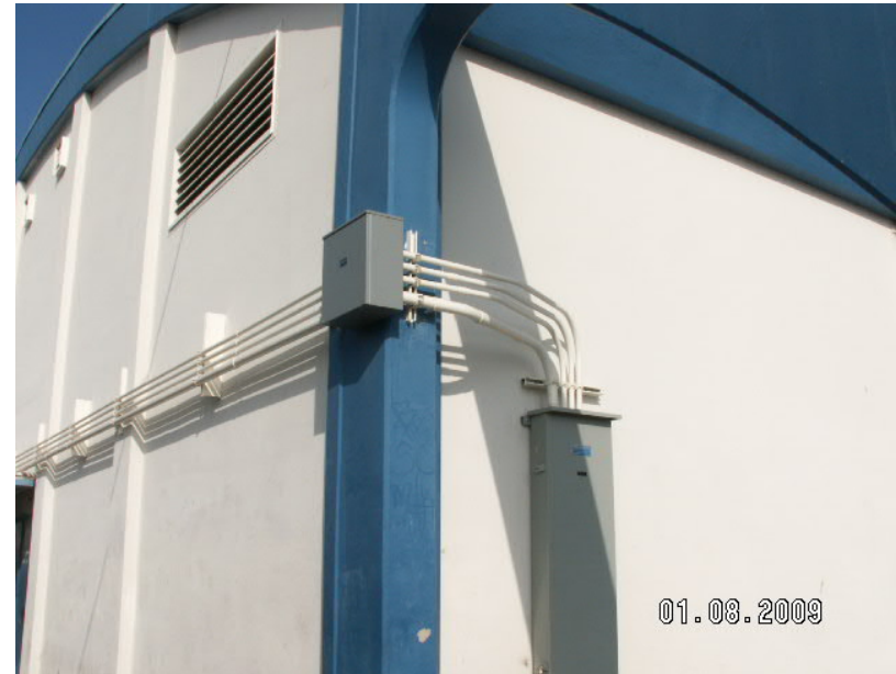
New power distribution conduits for the old GYM Building
