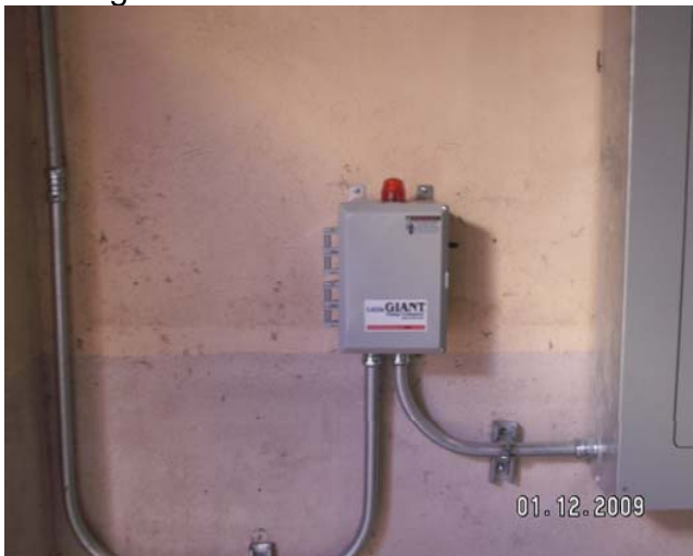
Duplex sump pump controller mounted inside
