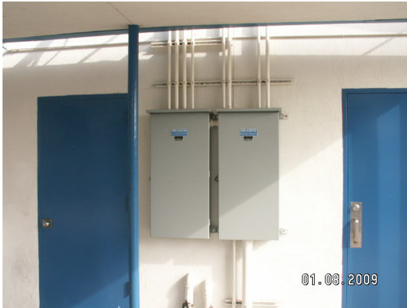
New power distribution panels on Building # 8 Typical of all the wing buildings
