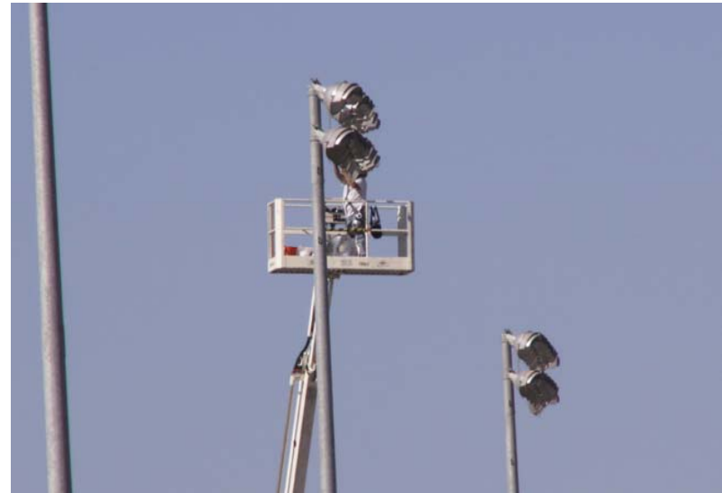
Replacing damaged reflector lens
