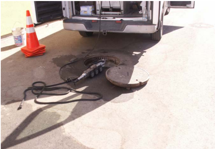
Inserting high resolution camera into sewer
