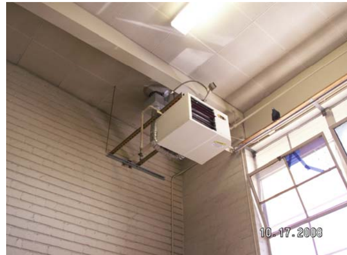
New Reznor Ceiling Units installed in classrooms
