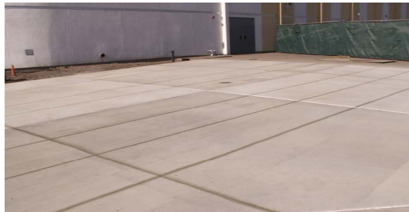
New concrete flat work with expansion joints
