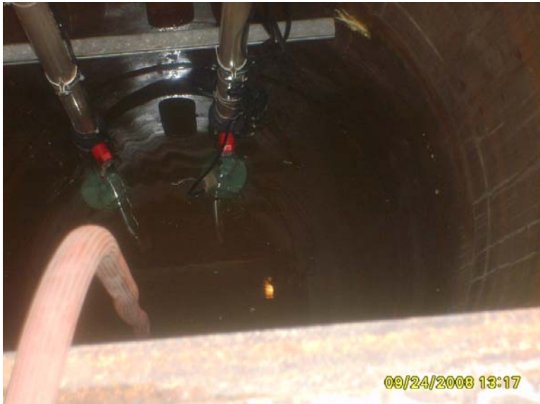
New Duplex Sump Pumps completed and “Rain” tested
