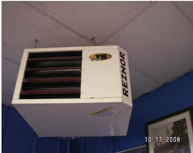
New Reznor Ceiling Units installed in classrooms
