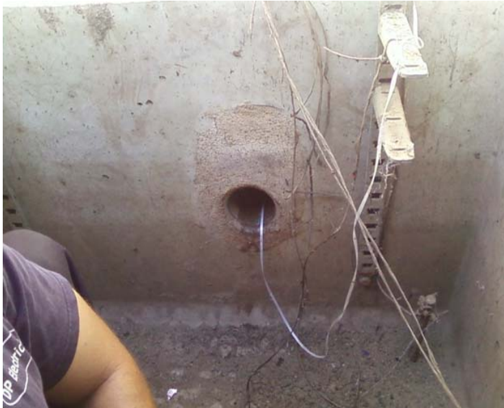
Running tape to determine length
