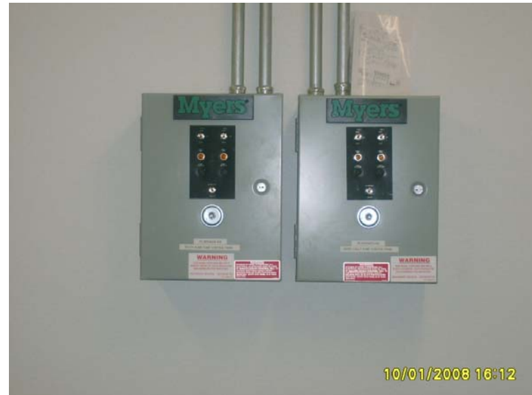
Newly Installed Sump Pump Controller Units
