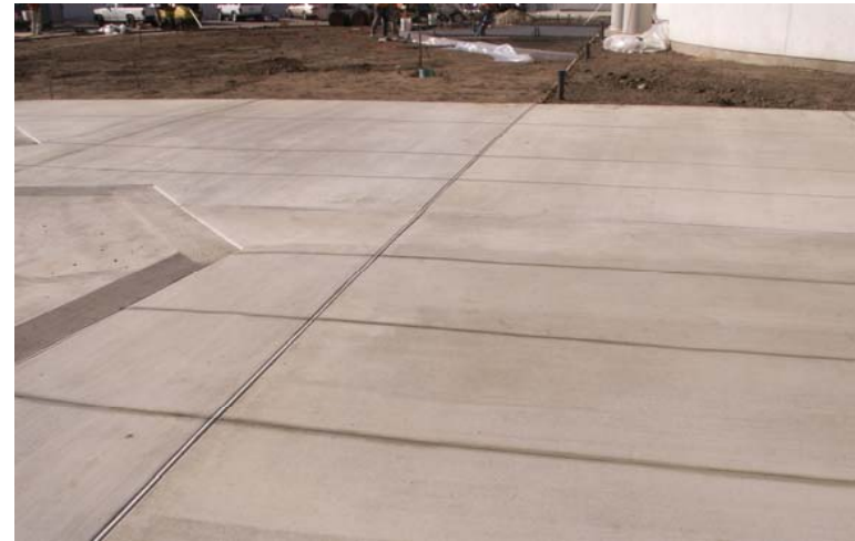
New concrete flat work prior to sand blasted finish
